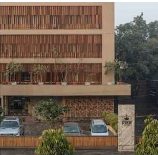
Client: Levana Hospitality LLP / Project Location: Lucknow, Uttar Pradesh, India / Built up Area: 3000 sq.mtr
